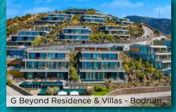
G Beyond Residence & Villas - Bodrum
